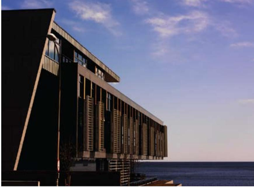
The granite serves as a “frame” around the main structure of the building, which also includes elements of metal and glass. The finishes are flamed and “Silk,” a matte-structured finish obtained by using abrasive tools from Tenax.
